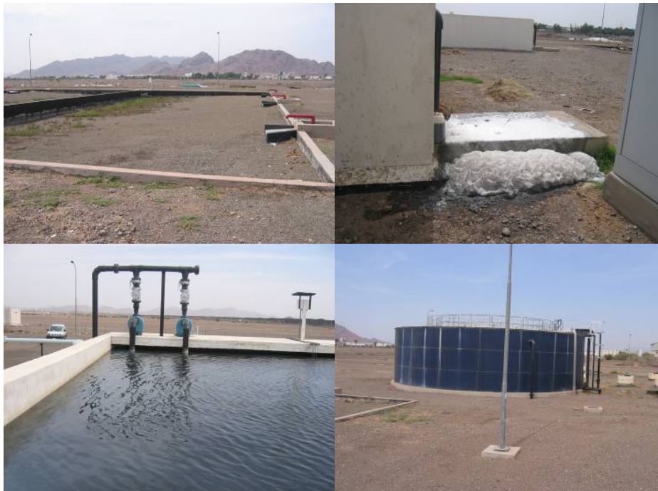
existing sewage treatment plant, proposed to be dismantled
